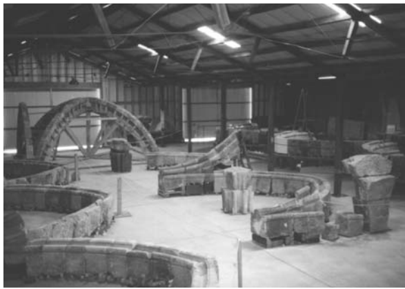
Arches are reassembled to determine exact placement of stones
